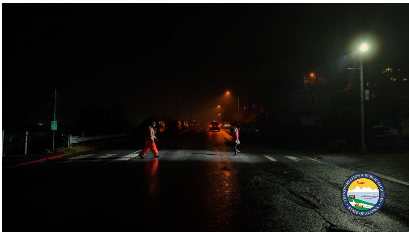
Figure 8: Soffit Light Installed at Kodiak Lighted Crosswalk
